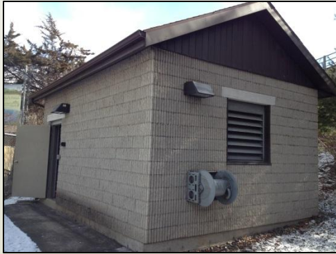
Pines Bridge Pump Station
