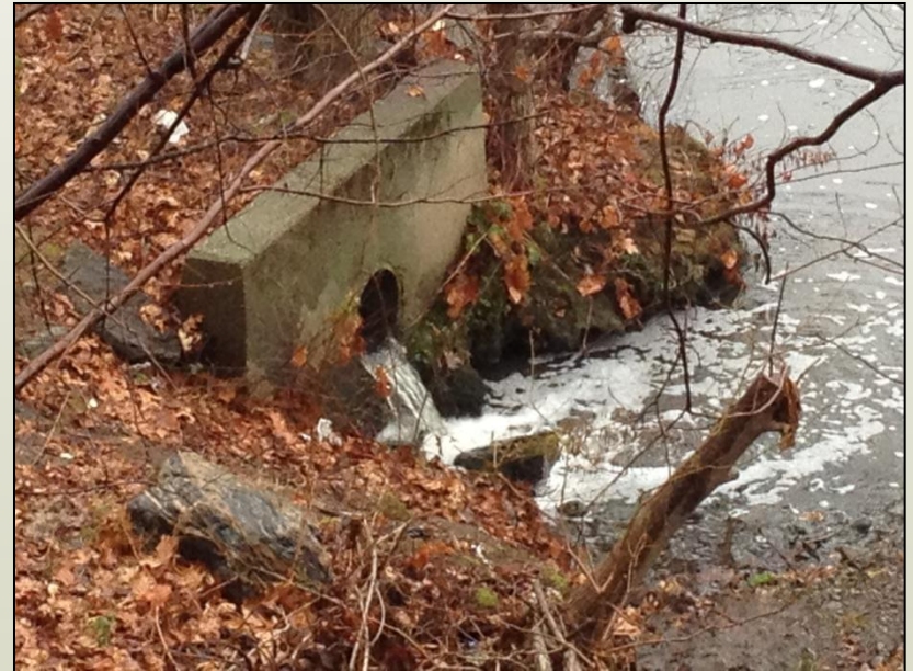
Beacon Falls WPCF Outfall @ Naugatuck River
